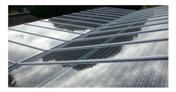
It was decided to go for the design of a roof with minimum inclination, capable of safely draining rainwater and at the same time versatile for any orientation, thus the location losses never exceed 8%.
